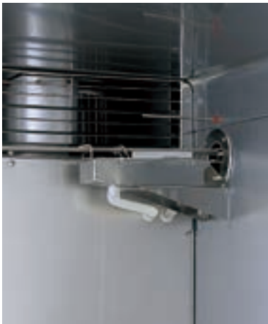
Wick installation (Test area)
